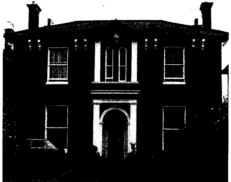
Grosvenor Road Community Residence in Rathgar, Dublin.
