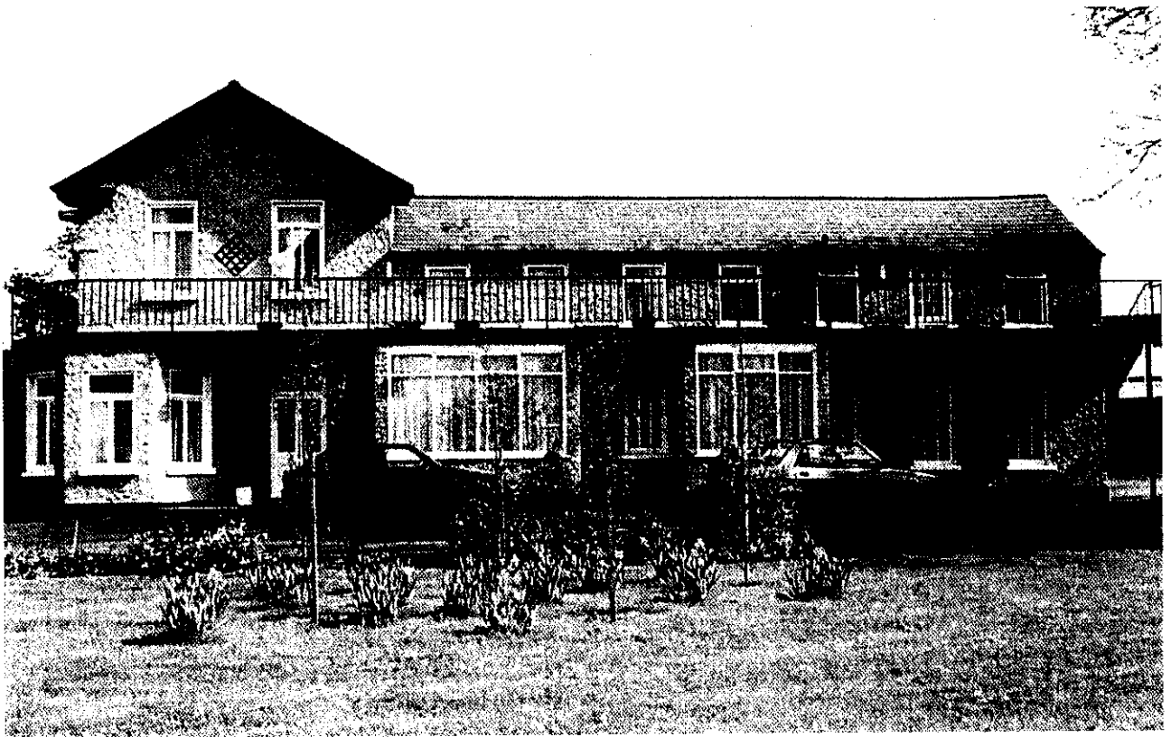
Community Residence, Grove House, Celbridge, Co. Kildare.
