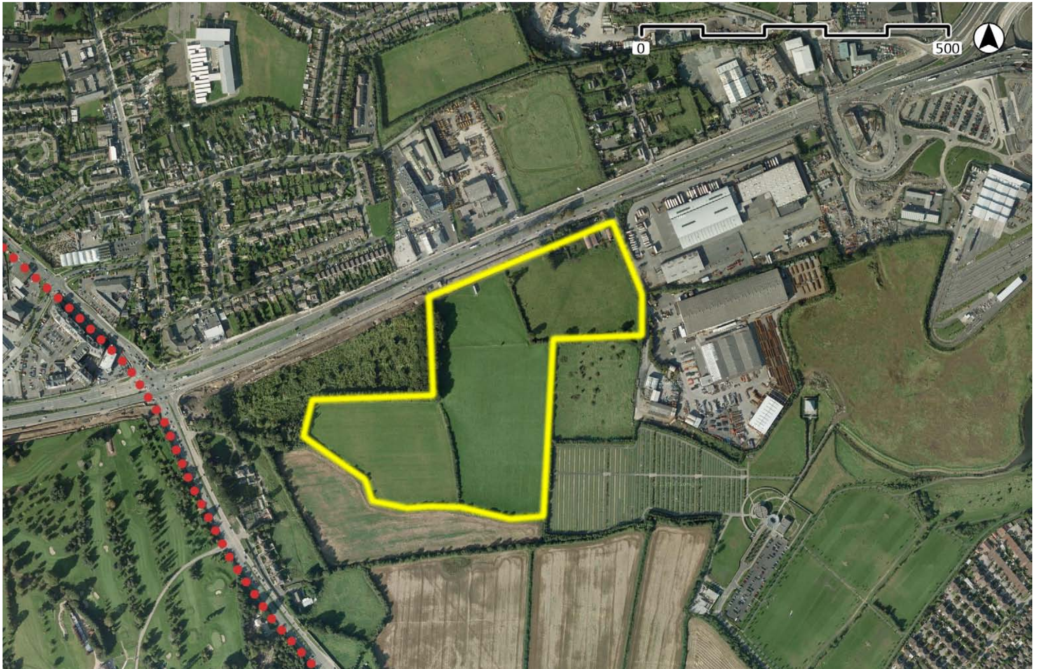
Aerial View Site B
