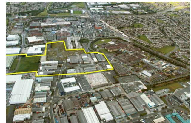
Aerial View looking SOUTH
